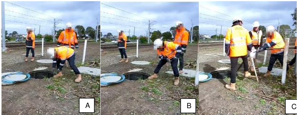
Figure 4. Cable pulling without(A and B) and with (C) the trestle
