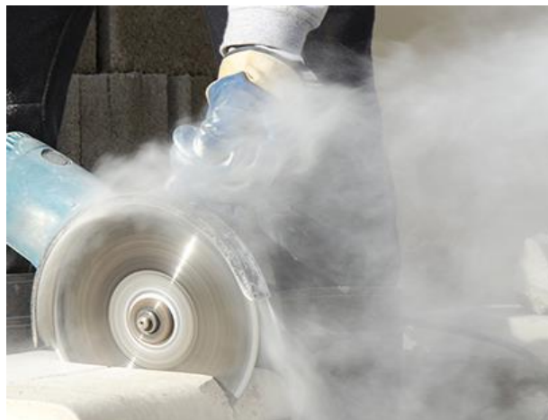
Figure 4 - RCS generation during stone benchtop cutting
